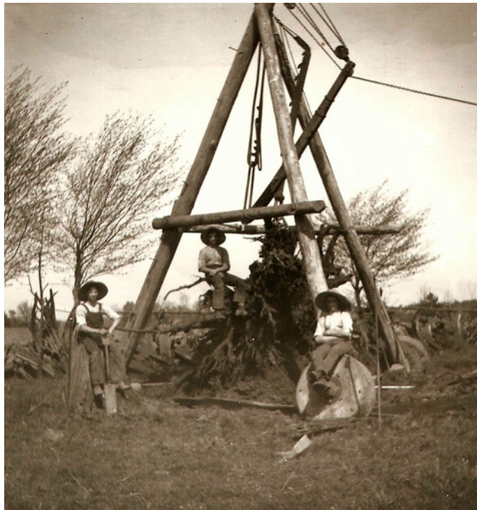
Fig 2 - Stump pulling on the Moore Farm EHS 14410.
